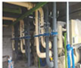
Piping Installation Work
