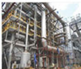
Structural Steel Pipe Rack
