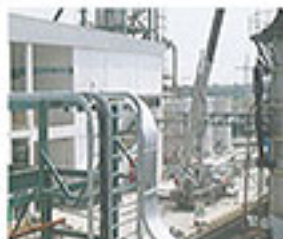
Structure Pipe Rack
