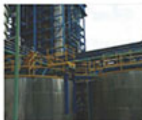
Stainless Steel Manufacturing Work
