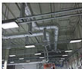
Exhaust Ductwork
