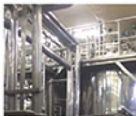
Plant and Piping Installation
