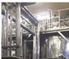
Plant and Piping Installation
