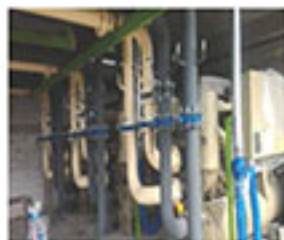
Piping Installation Work
