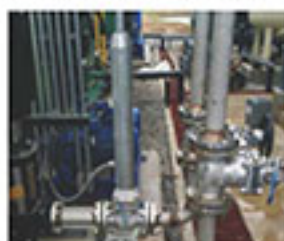
Industrial Piping Work
