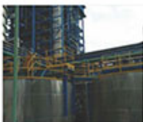
Stainless Steel Manufacturing Work
