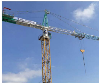
Tower Crane Potain ម៉ាក Topkit MD 238-12
