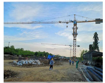
Tower Crane Potain ម៉ាក SP 175
